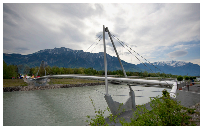
Buchs-Schaan Energy Bridge – one of Liechtenstein's flagship projects.
