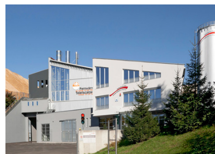
District heating power plant in Brunico
